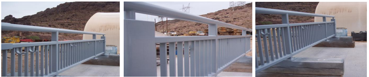
Railings were power washed at 3,500 psi and primed with Rust Grip®.
